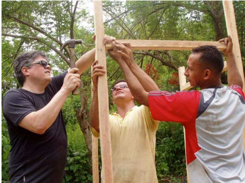
Building a latrine during UUCC's 2014 Honduras Service Trip
